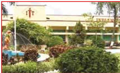
UNIT NO.1 NASIK PLANT
